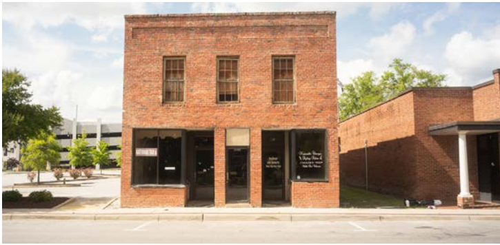
Downtown Florence Retail Accelerator Site
