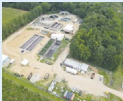
Wastewater treatment plant and lab - Upgrades to the wastewater treatment plant include the finished construction of two new aeration basins (left) and a new water testing lab that is nearing completion.
