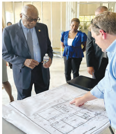
John Hendrix, director of Construction with G.M.K. Associates, shows Congressman James E. Clyburn and Lake City Mayor Yamekia Robinson architectural drawings detailing the renovations at the future community center under construction on Cole Road in Lake City. The congressman visited Lake City Aug. 9, for a working lunch and tour of the community that detailed progress and plans for future growth.
