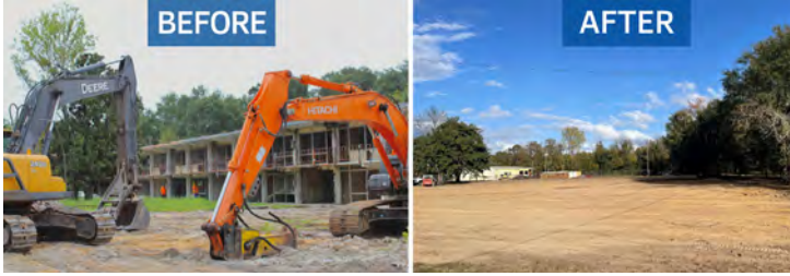
Home Demolition at 408 Johns Street
