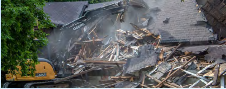
408 Johns Street Demolition Progress
