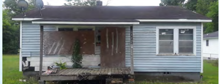
112 East Liberty Street - Before Demolition
