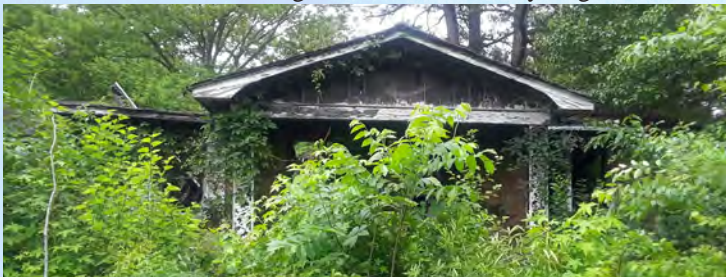
1102 Harmony Street – Before
