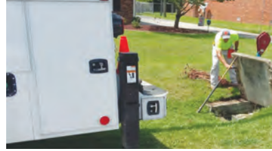
Work for the Stormwater Capital Improvement Program
