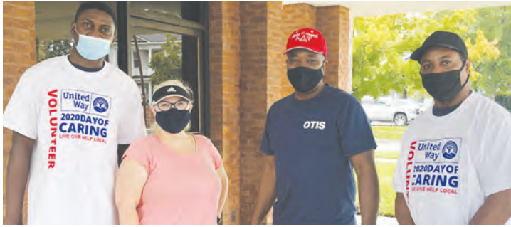
Volunteers from Otis Elevators helped paint, pressure wash, repair and landscape at Mercy Medicine Free Clinic for our 28th Annual Day of Caring.
