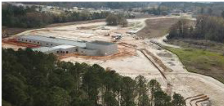
Aerial view of construction at the new school location
