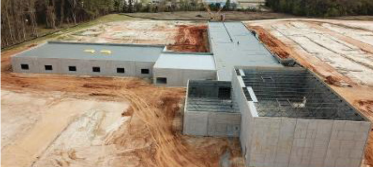
View of the new school under construction and work on the interior of the building has begun.
