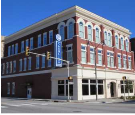
Carolina's Bank new downtown location
