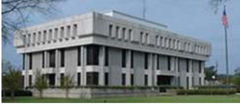
City of Dillon Administration Building
