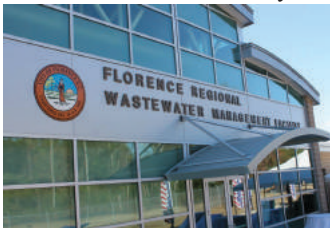
Waste Water Management Facility
