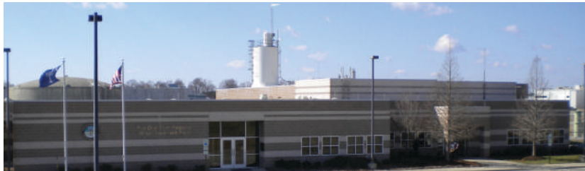
Pee Dee Regional Surface Water Treatment Plant
