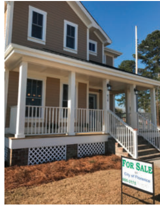
Vista Place House 414
