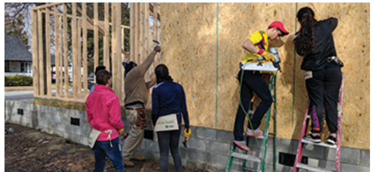
GSSM Students helping to build the new home
